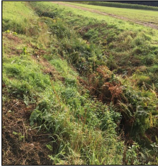
Photograph 7: Dry Ditch between Fields F9 and F7 (September 2017)
