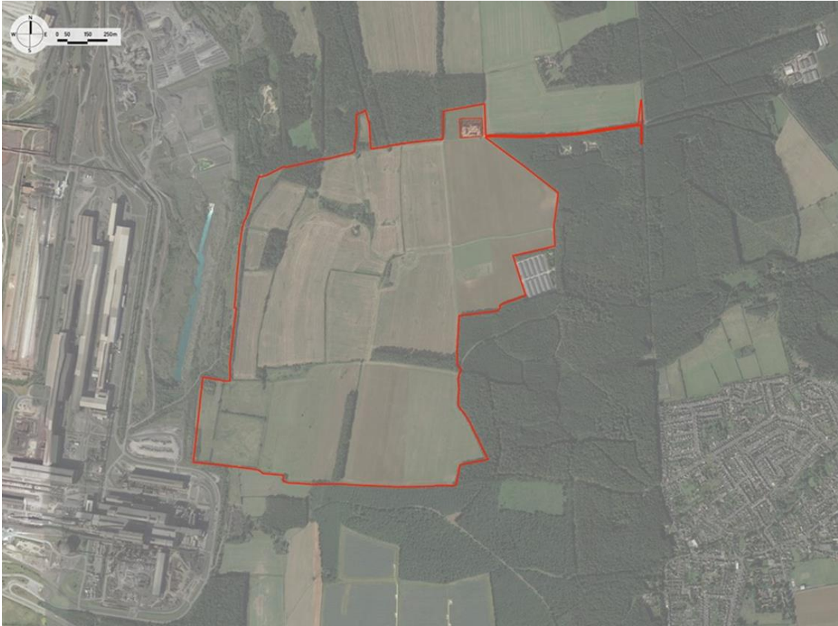
Figure 2: Aerial photograph of Order Limits
